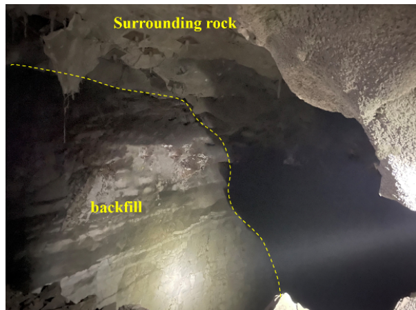
Fig. 1 – The backfill supports the surrounding rock
