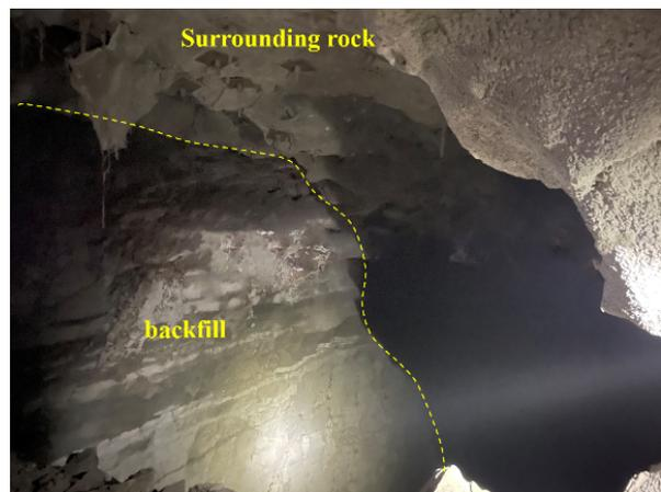
Fig. 1 – The backfill supports the surrounding rock
