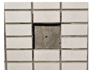
1) Removed Tiles 2) Wall Surface after Tile Removal
