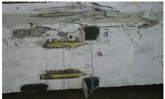
(f) concrete crushing at top at ultimate load
