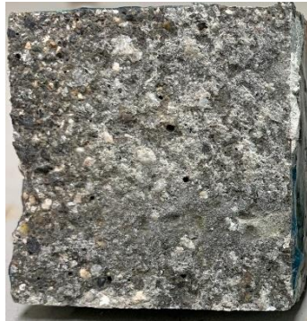
(a) Interface failure
