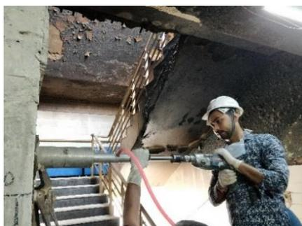
Fig.13 – Extraction of concrete core from column of fire damaged floor
