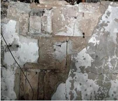
Fig. 4 – Excessive cracking and damage in foam concrete blocks
