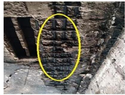
Fig.9 – Spalling of concrete due to corrosion
