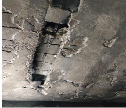
Fig. 5 – Spalling of ceiling plaster
