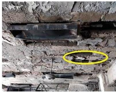
Fig.8 – Delamination of cover concrete in the cross beams
