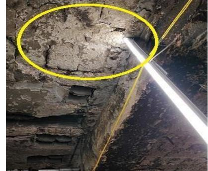
Fig. 6 – Damaged hollow concrete blocks of the ceiling
