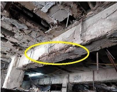
Fig.7 – Spalling of concrete in bottom edges of the main longitudinal ceiling beams
