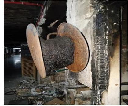
Fig. 3 – Melting of Rubber hose pipe of fire hydrant
