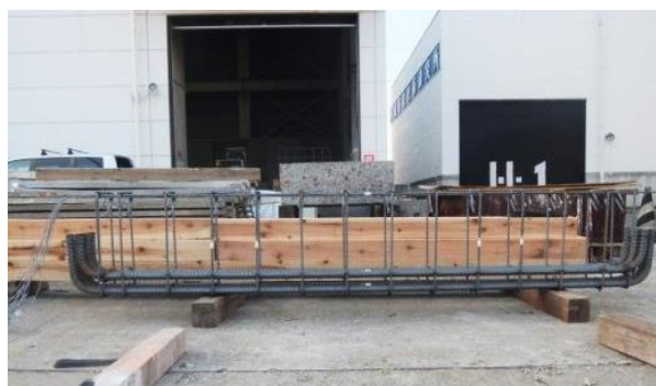
Fig. 3 – Reinforcing bars and stirrups
