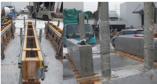
Fig. 5 – RC beams fabrication
