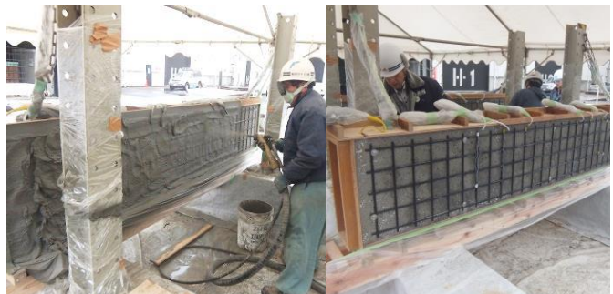
Fig. 6 – Fixing CFRP grid and spraying mortar
