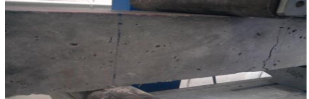
Fig. 17 – KFRC prism failure
