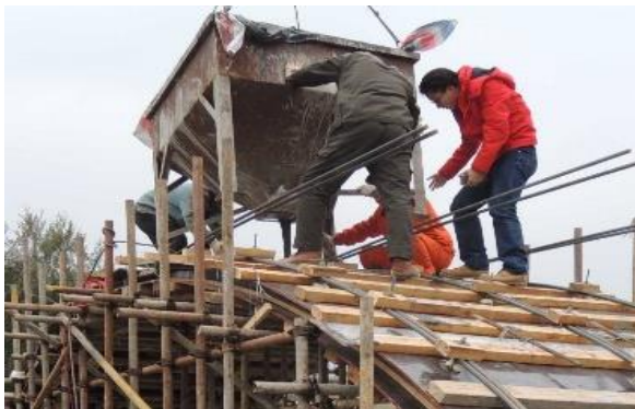
(a) Under construction
