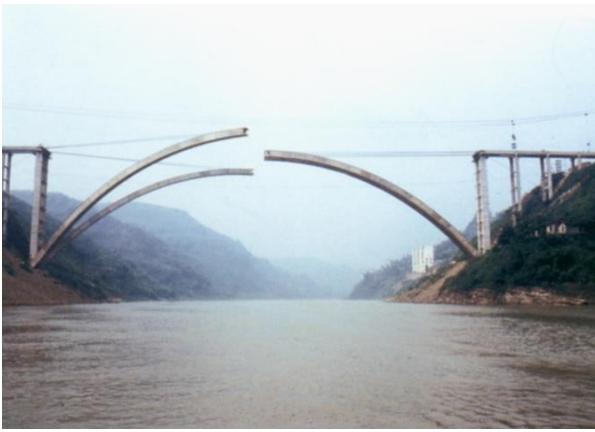
Fig. 6 – Horizontal Swing method in Fuling Bridge in Sichuan
