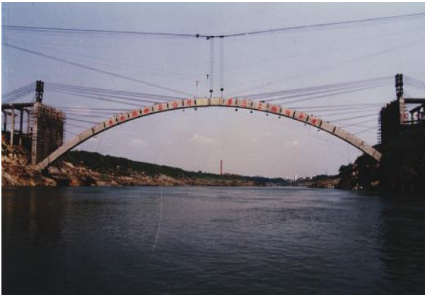
Fig. 4 – Cantilever assembling method in the Moding Bridge in Guangxi
