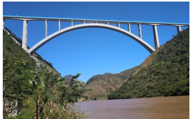
Fig. 3 – Nanpanjiang Railway Bridge
