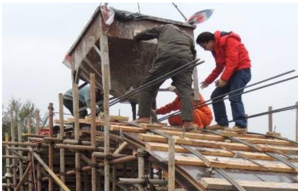
(a) Under construction
