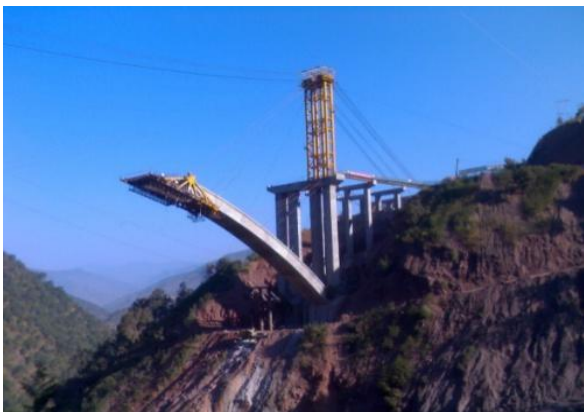
Fig. 5 – Cantilever cast-in-situ method in the Baishaguo Bridge in Sichuan
