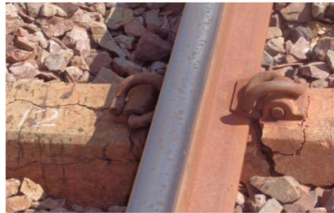
(c) Failure cracks observed at the location of the insert in the concrete sleepers
