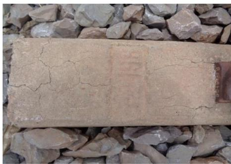
(a) Map cracks observed at the end of the concrete sleepers
