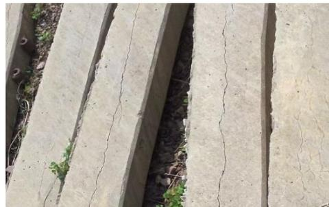
(b) Longitudinal cracks observed at the middle of the concrete sleepers
