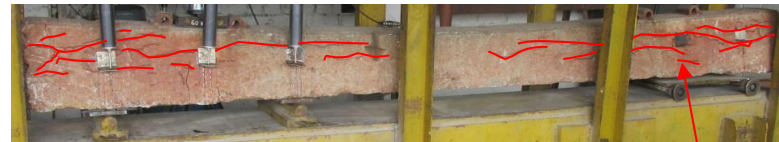
b) Severe Damaged Sleeper 3 mm cracks
