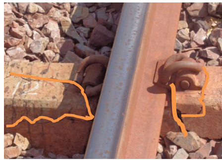
(c) Third Step (Cracks near insert location)
