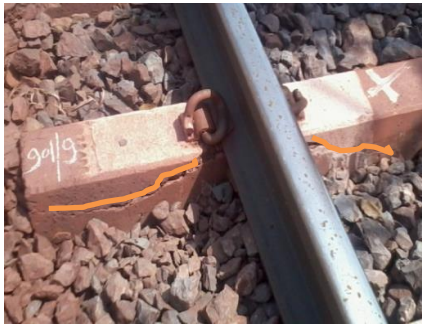
(c) Third Step (Cracks near insert location)
