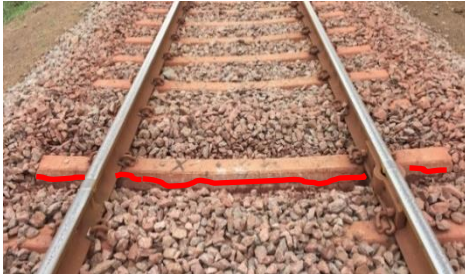
(a) First Step (Cracks at side face) (b) Second Step (Cracks visible on top surface)
