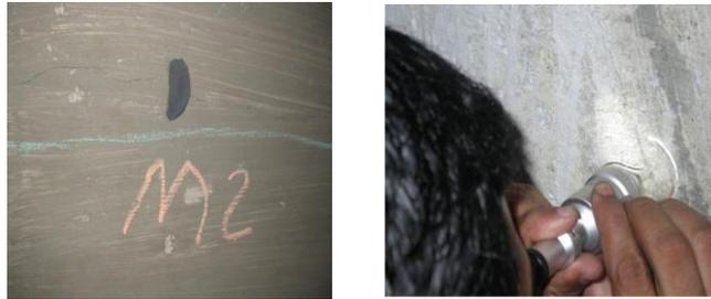
Fig. 1 – Crack measurement on upstream and downstream side of upper gallery-3
